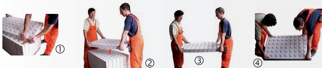
First lower the VarioComp panels onto one edge and then lower them completely. Vertical storage leads to deformation of the panels and damage to the edges. It is possible to transport the panels horizontally inside the building with a lift truck or other panel transportation vehicle.
