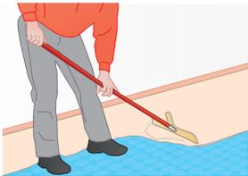
After 3 hours have passed (at 20 °C) after adding the VarioComp filling compound the surface of the VarioComp system must be primed (for product examples see chapter 5.4). Then, the second layer of VarioComp filling compound is applied.
