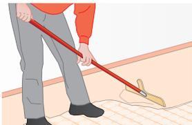
Within 3 hours (at 20 °C) after adding the VarioComp filling compound a 2nd layer of VarioComp filling compound is applied.
