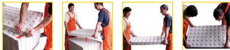
First lower the VarioComp panels onto one edge and then lower them completely. Vertical storage leads to deformation of the panels and damage to the edges. It is possible to transport the panels horizontally inside the building with a lift truck or other panel transportation vehicle.
